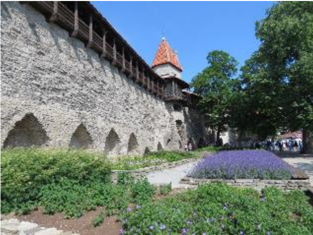
Tallinn walls with walkway on top.
