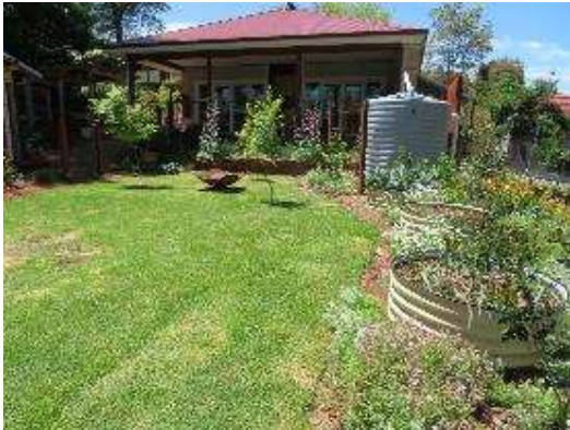
Figure 13 Dairy Lane Cottage
